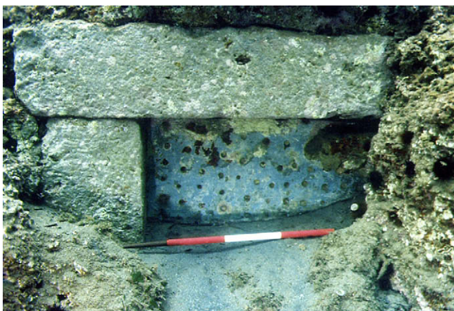
Fig. 3. Ventotene fishpond: the fixed sluice gate (Lambeck et al., 2004b).
