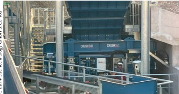
Installation Primary Crusher DRC 900-20
