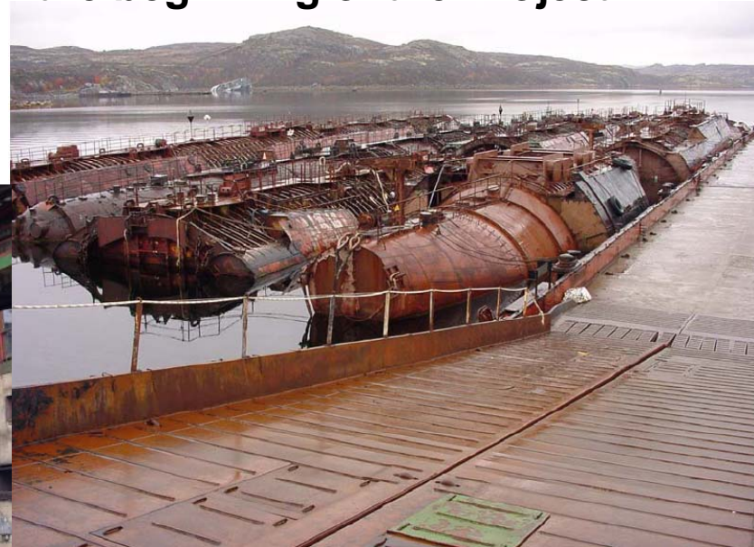
Situation at the Sayda Bay at the beginning of the Project
