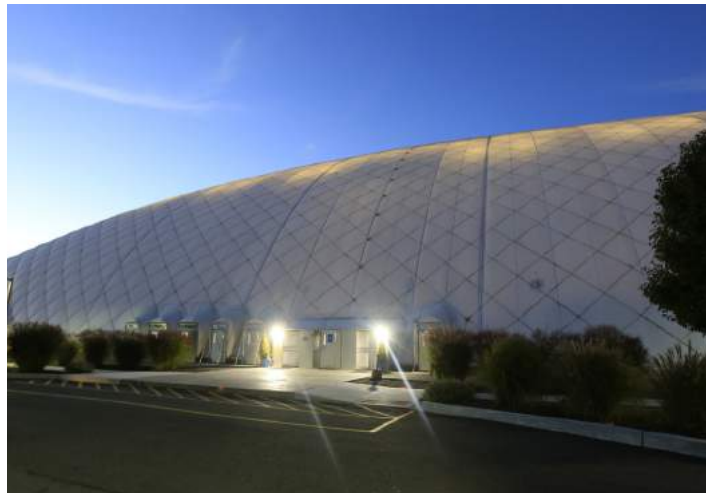
Alioth Ultra wall packs brightly illuminate the entrance to the dome.
