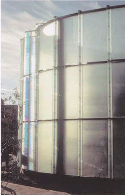
James Carpenter Design Associates, United States Glass Scrim Wall , Scottsdale Museum, Phoenix, Arizona, 1999 Rebecca Uss and Aki Ashida, project architects; William P. Bruder, museum architect Photo: James Carpenter, courtesy of James Carpenter Design Associates, New York, New York DC
