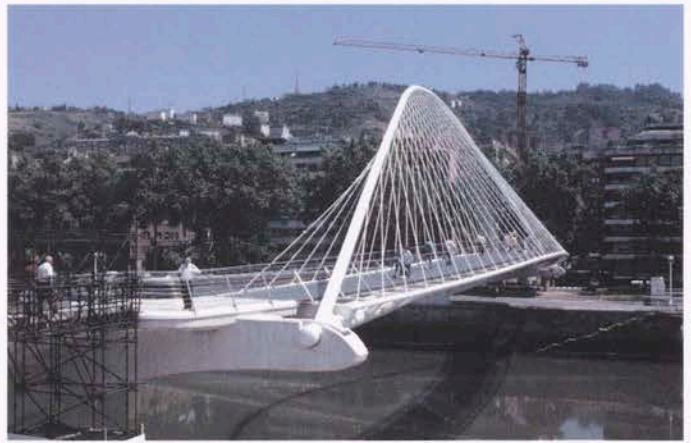
Santiago Calatrava, Spain Campo Volantin Footbridge , Bilbao, Spain, 1990–1997 Steel inclined parabolic arch; glass decking Geneigter stählerner Parabolbogen; Glasbedachung Photo: GreatBuildings.com Photo © Artifice Inc., Eugene, Oregon DC
