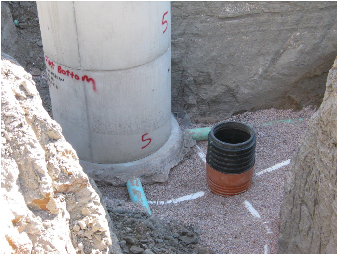
Example of a typical inspection pit installation
