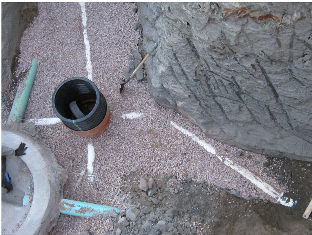
Example of a typical inspection pit installation
