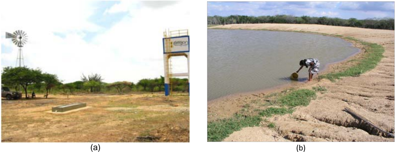
Photo 4. Water supply systems of Wayuu rural settlements
