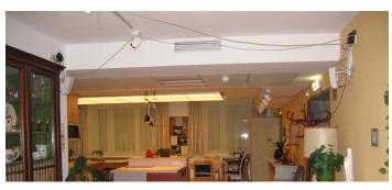
(a) Sensor installment in the living room. Provisional additional wires between the Ubisense Sensor Beacon were needed.
