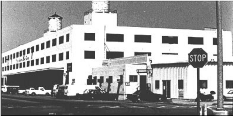
■ Figure 5.24 Building 116, Naval Supply Facility, San Diego
