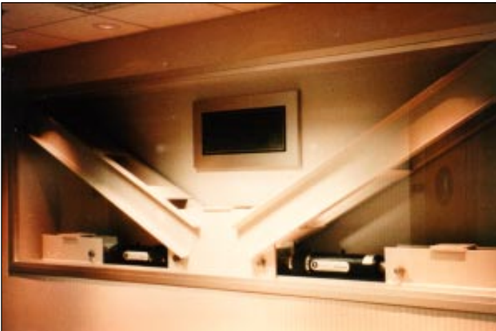
■ Figure 5.32 Damper Installation in the Pacific Bell North Area Operations Center
