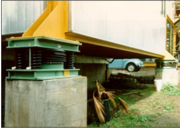
■ Figure 5.27 Spring and Viscous Damper System in Small Residential Building in Los Angeles
