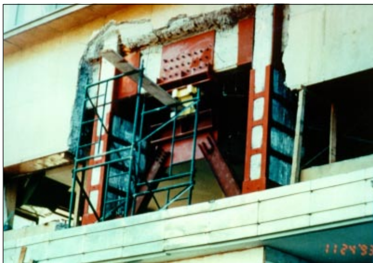
■ Figure 5.5 Brace-Damper IMSS Reforma Building Retrofit Scheme from Outside
