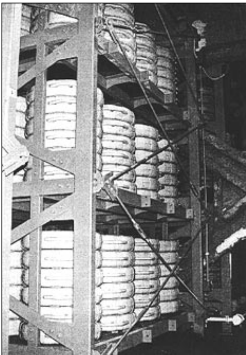
■ Figure 5.44 Installation of Vessels in TLD Room in Tower
