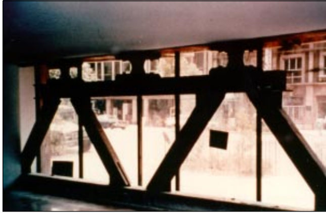
■ Figure 5.2 Brace-Damper Assembly in Izazaga #38-40 Building
