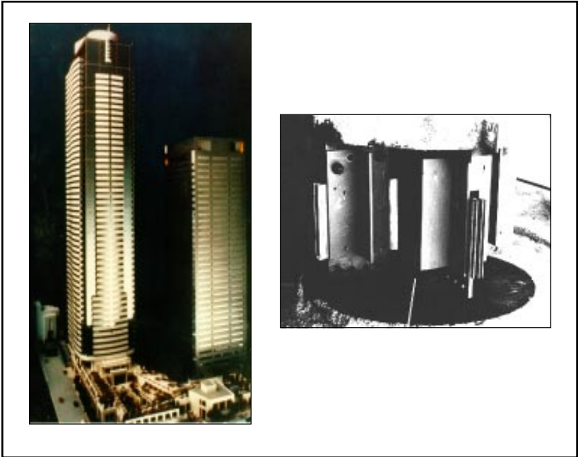
■ Figure 5.20 Damper Installation in the Two Union Square Building, Seattle
