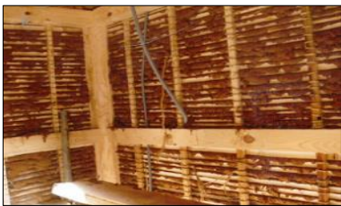
<Bamboo structured walls of a thatched house>
