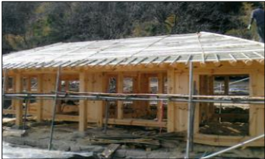
<Bamboo structure of a thatched house>
