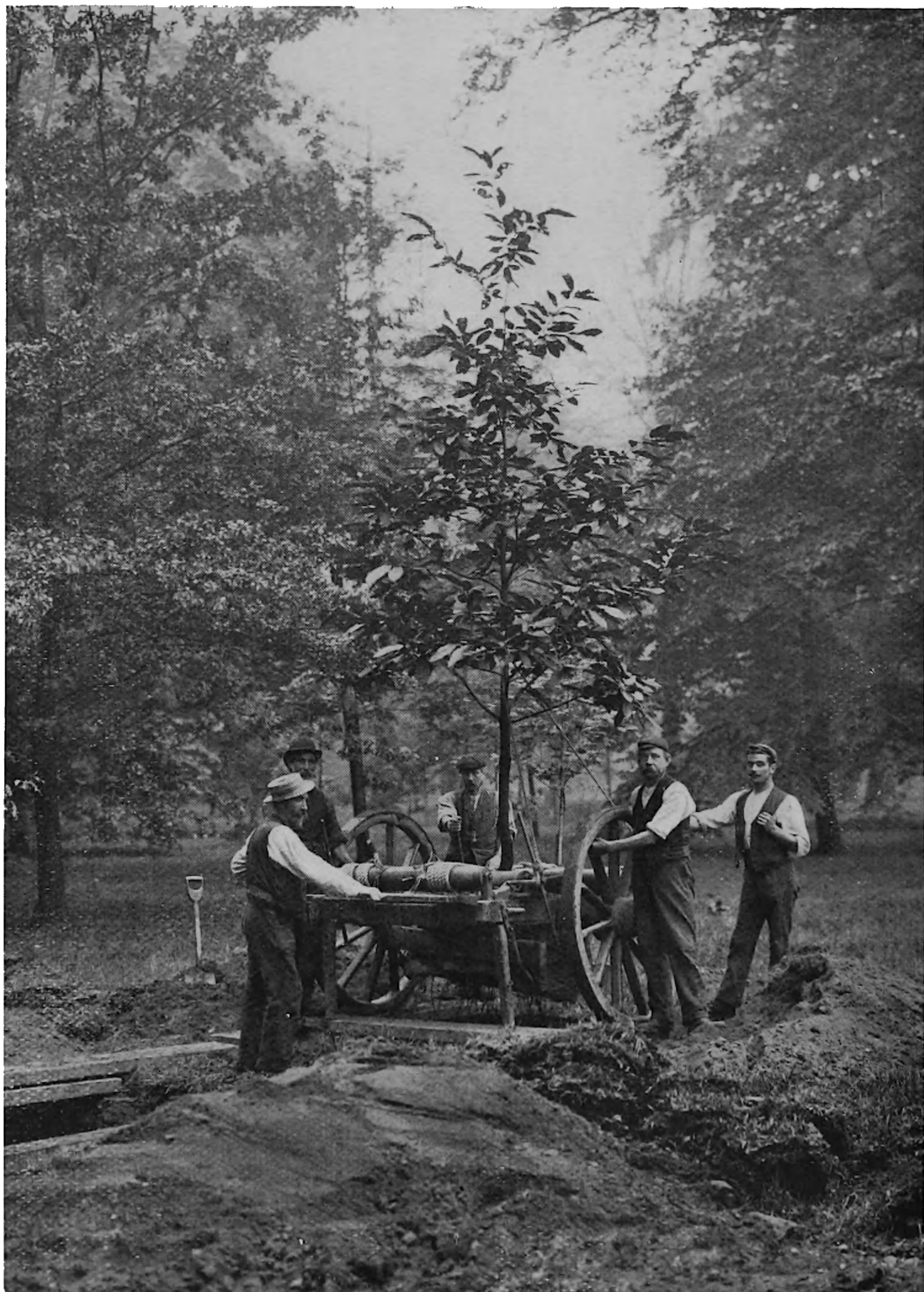
TREE IN COURSE OF REMOVAL WITH ONE OF BARRON'S MACHINES.
