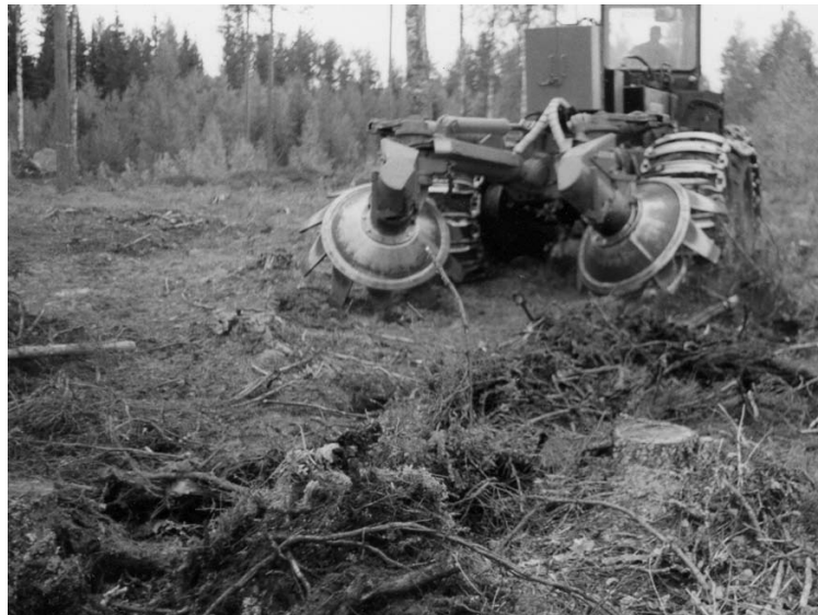
Fig.1. TTS Delta active disk trencher in work in the South of Finland.
