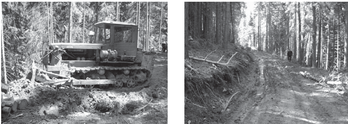
Fig. 12: Making of forest truck roads for timber transporting
