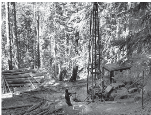
Cable way system "TBC - 500 (TVS-500)"
