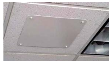
Installed antenna fits flush with ceiling.
