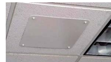
Installed antenna fits flush with ceiling.
