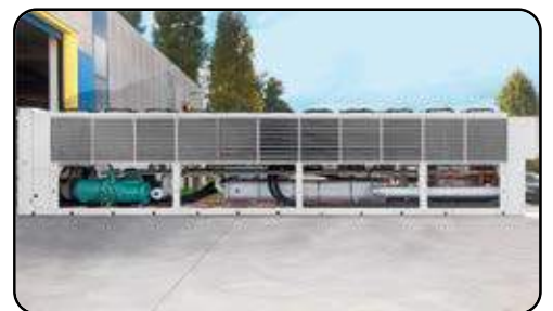
Free-cooling chiller, 1240kW * 460/3/60 UL, ASME evaporator Installed in USA for Data Center
