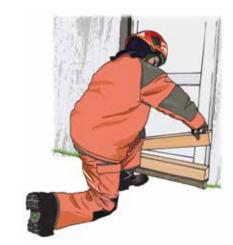
Now select the appropriate struts and extensions for the measured space and assemble two shores of the same length.
