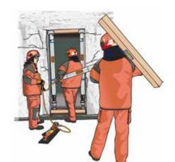
This type of shore should be assembled in a safe area and then moved into place. They are normally installed with wood above and below to spread the load.
