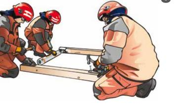
Now that the shores are assembled, nail the heads to either end of the wood header ensuring the shores remain parallel.
