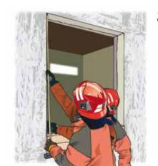
After placing the header and footer on top of each other in the opening, measure the length of shore required.
