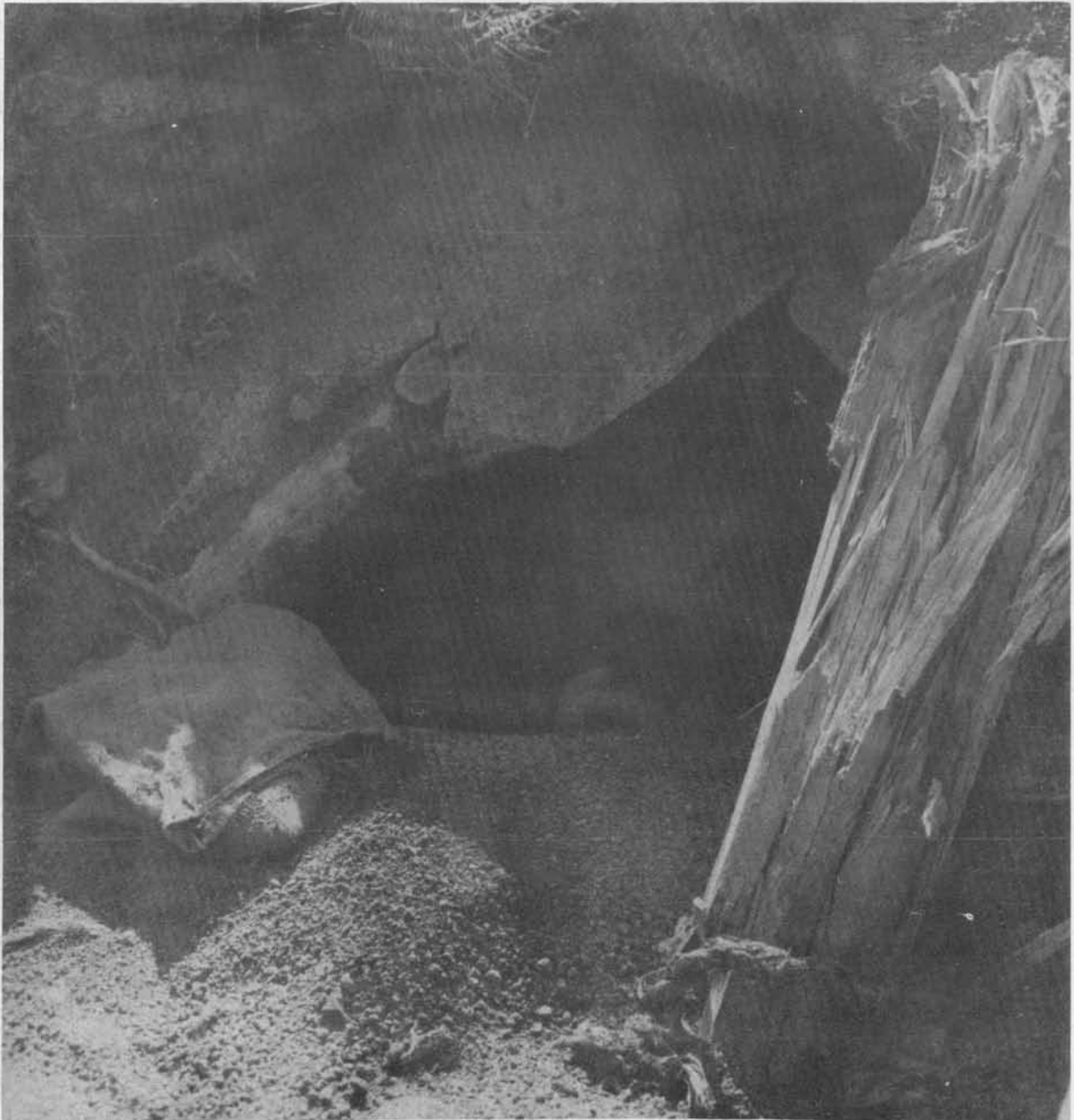
ENTRANCE TO DAMAGED PILLBOX BETWEEN BEACHES RED ONE AND TWO Construction was of logs and concrete covered with sand.
