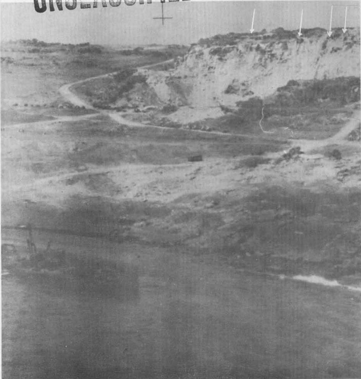
BATTERY OF FOUR CASEMATED GUNS IN CLIFF AREA (Photo--February 3, 1945)
