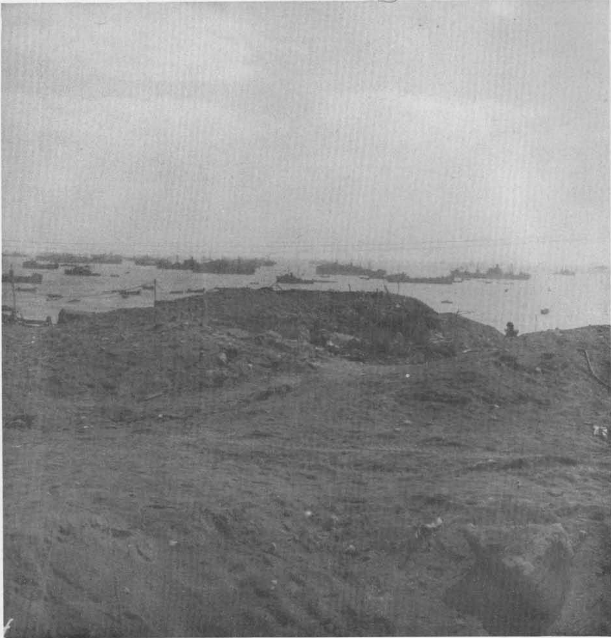
TARGET 114 Damaged blockhouse YELLOW Beach ONE
