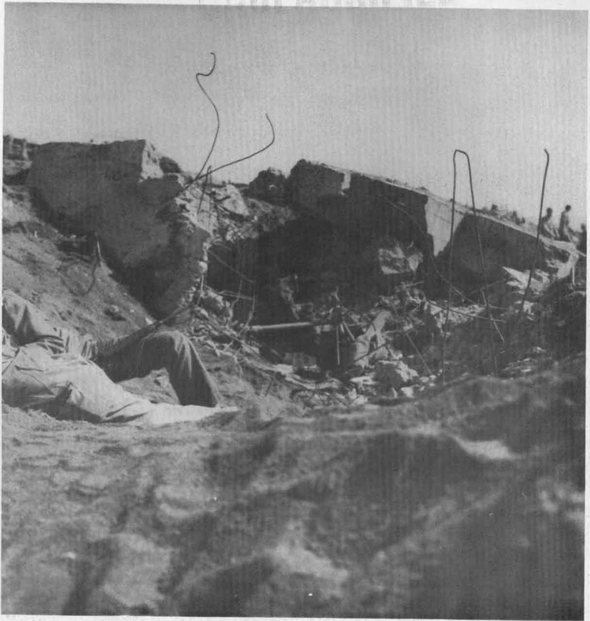
WRECKED BLOCKHOUSE - RED BEACH ONE Concrete slabs used in blockhouse construction were 24 to 48 inches thick.
