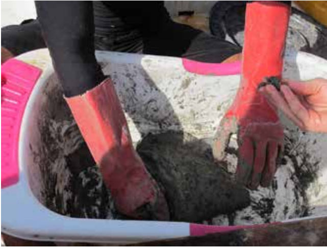
Figure 36. Mixing the cement on the boat.
