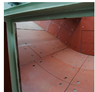
Replacement liner plates within the submerged ash extractor
