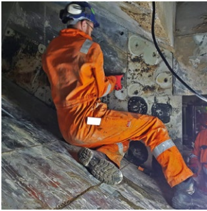
Removal of worn liner plates
