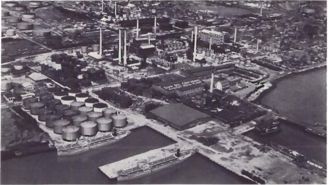
Air view of Sun Oil Company Refinery, Marcus Hook, Pa. Kingsbury Thrust Bearings are used in the multi-stage centrifugal pumps by which hot oil, under high pressure, is moved through the refining processes. They are used also on the propeller shafts of the ocean and river tankers, some of which are seen in the foreground.
