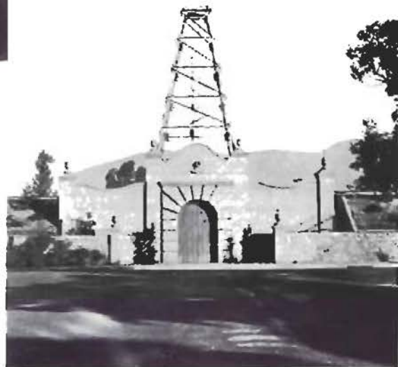
Right: Villa Street Pumping Plant, Pasadena Water Department, Pasadena, Calif. The deep well centrifugal pumps use Kingsbury Thrust Bearings.
