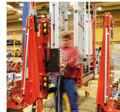
Cabling of sensors
