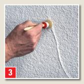
Depending on the texture of the decorative plaster, adapt fresh sealant to the surface of the plaster using a brush or trowel.
