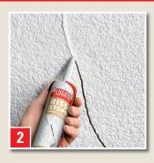
Inject RISS-STOPP into the crack with a sealant gun.
