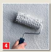
Allow the RISS-STOPP to dry and coat with emulsion paint, for example.
