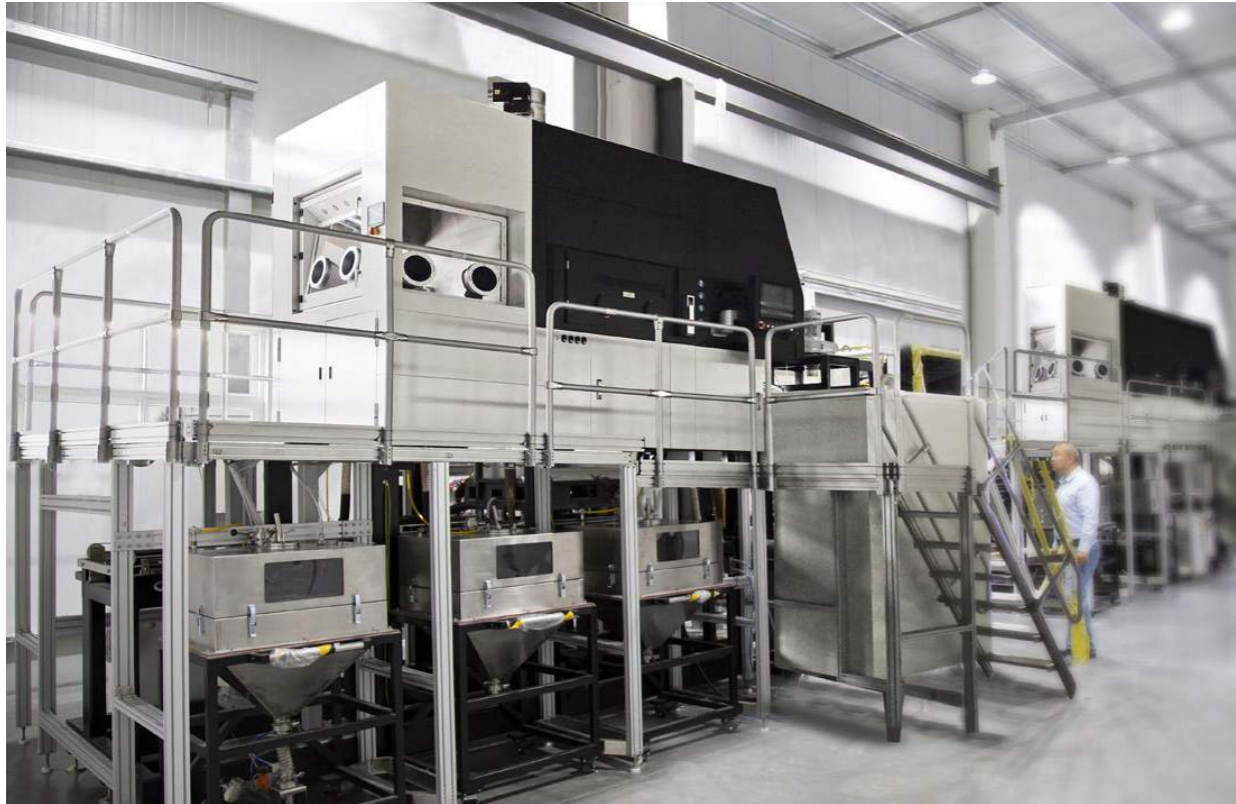
Fig. 7 Multiple FS621M system installed at Falcontech Super AM Factory (Courtesy Falcontech)
