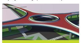
A striking, elevated traffic circle will be built at the intersection of Govan Mbeki Road and Jan Smuts Drive, where various MyCiTi routes will meet. The first of its kind, the 'Sky Circle' is designed to provide buses with uninterrupted travel across the intersection, without delaying traffic below.
