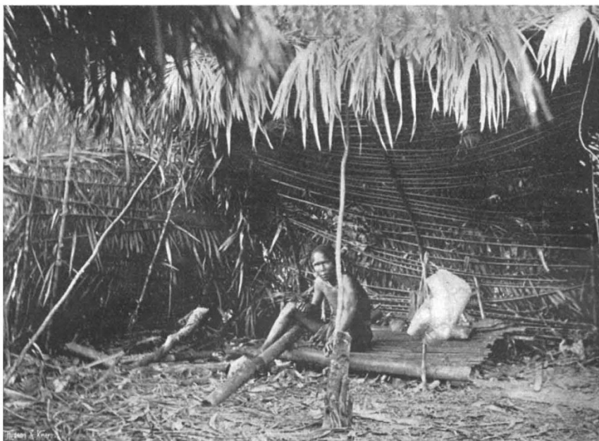
FIG. 1.—Semang (Semán) shelter, with kitchen (occupied by married couple); Grit, Upper Perak.
