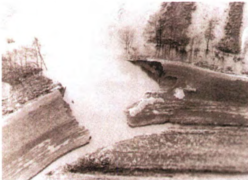
Figure 6.2-2. Photograph of Elba River bank breach in 1976 (Nagy, 2006)
