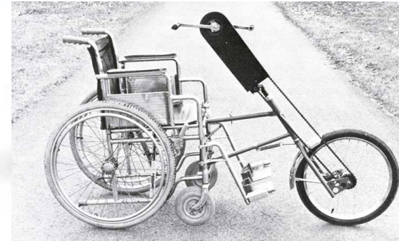
1983 - first attachable handcycle for a wheelchair.
