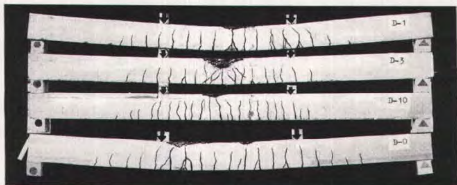
Fig. 9. Crack patterns at failure for beams of Group D.
