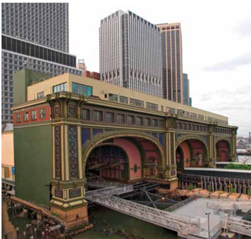
Staten Island Ferry Terminal
