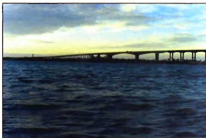
Bridge connecting Pamban & Rameswaram
