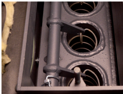
Fig. 7: Coupled turbulator
