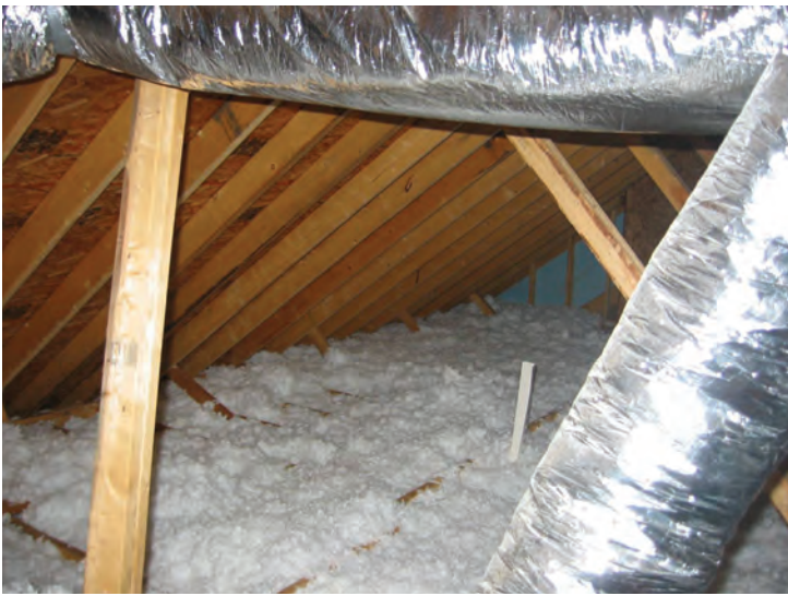
Figure 7.2. Blown Attic Insulation
