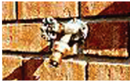
Figure 9.17. Hose Bib With Vacuum Breaker
