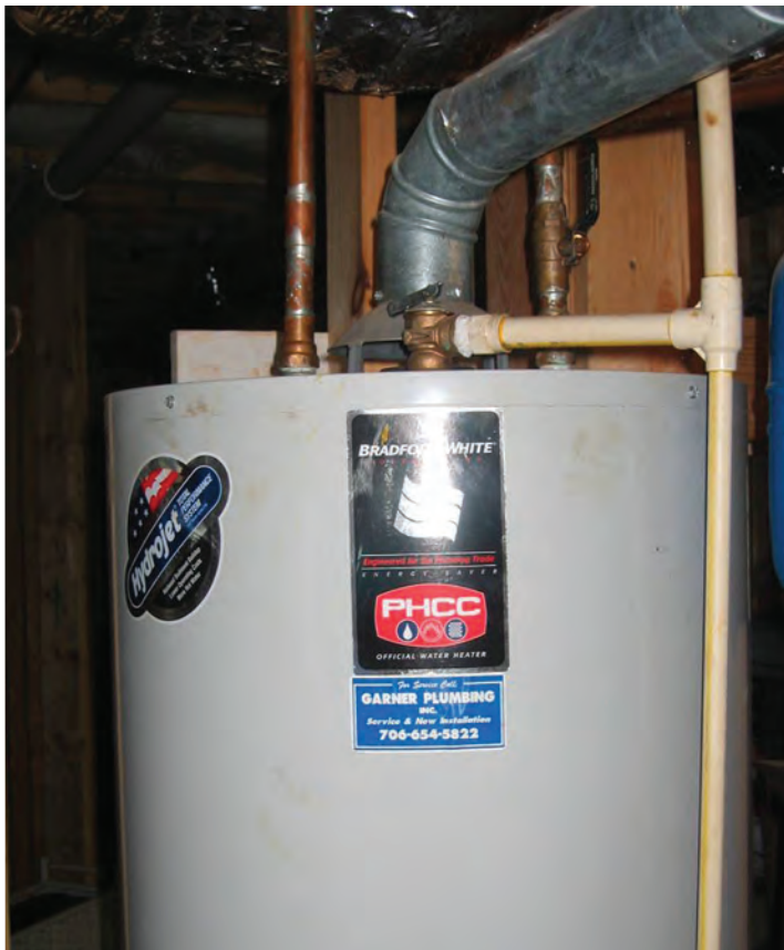
Figure 9.4. Temperature-Pressure Valve
