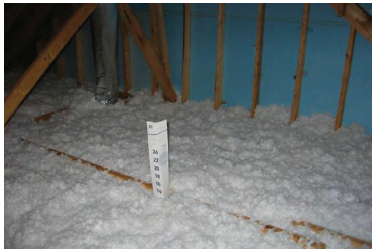
Figure 7.3. Depth of Attic Insulation
