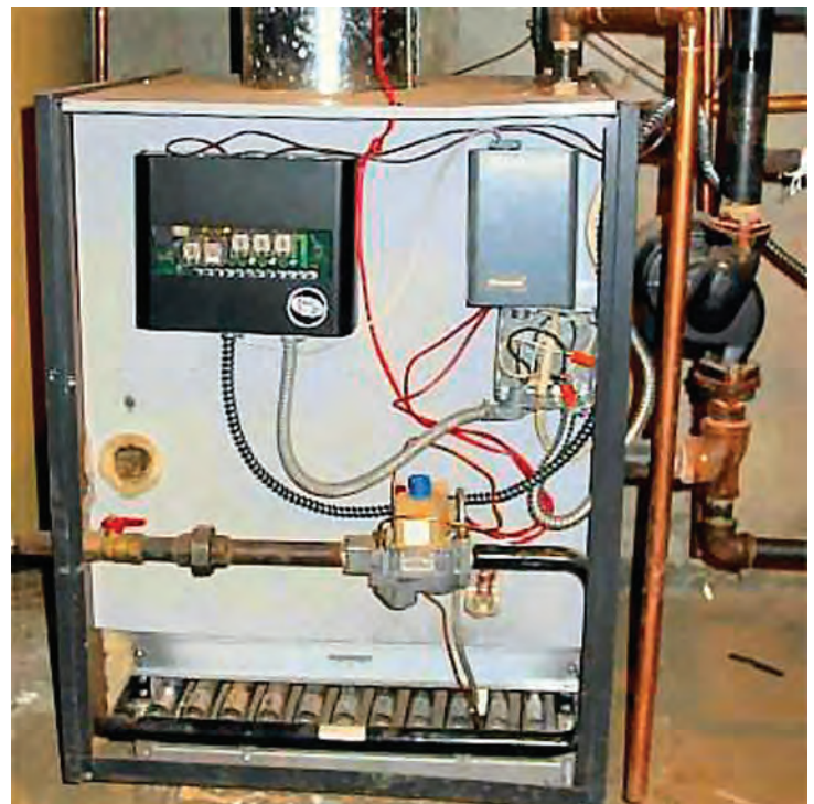
Figure 12.9. Gas-fired Boiler Source: HUD
