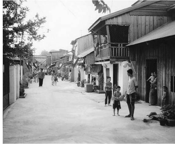
◀ Photo 7 / Photo 8: Before and after: Here are two photos of the main street in Ros Reay, Phnom Penh, before the improvements and after, with the drains and road and planting strips in place.
