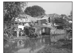
Figures 4 - 7 Flooding in 2007
