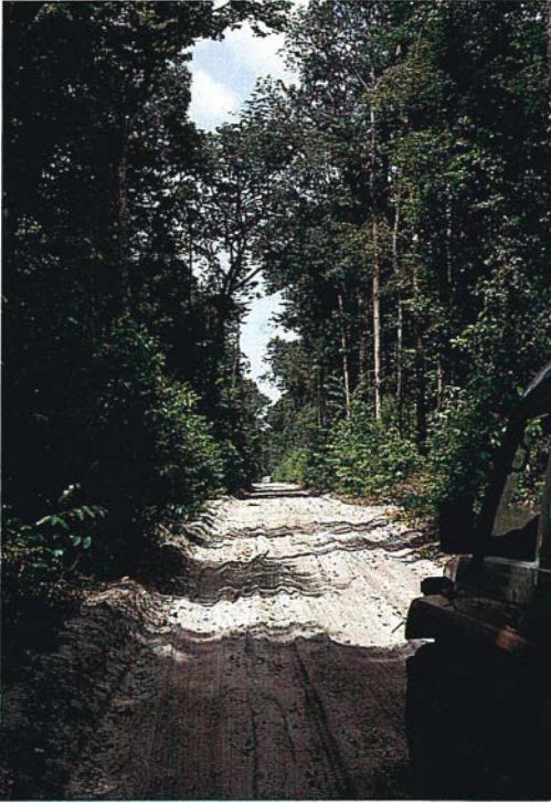
A small white sand road on top of a watershed is cause for little erosion problems.
