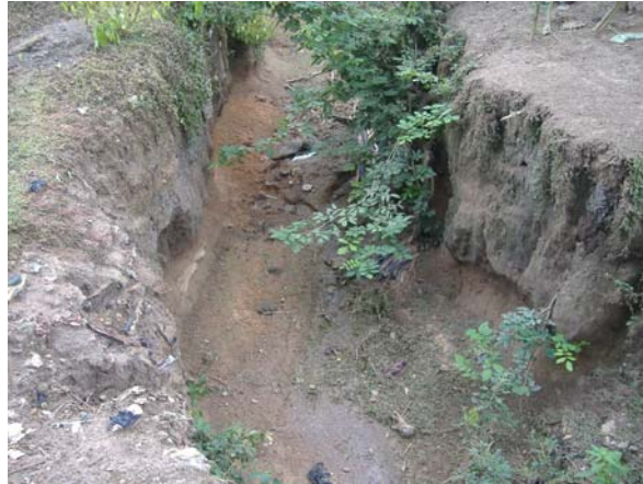
Gullies of this nature harbor mosquitoes in the rainy seasons.
