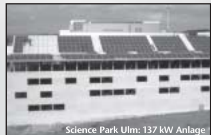
Science Park Ulm: 137 kW Anlage
