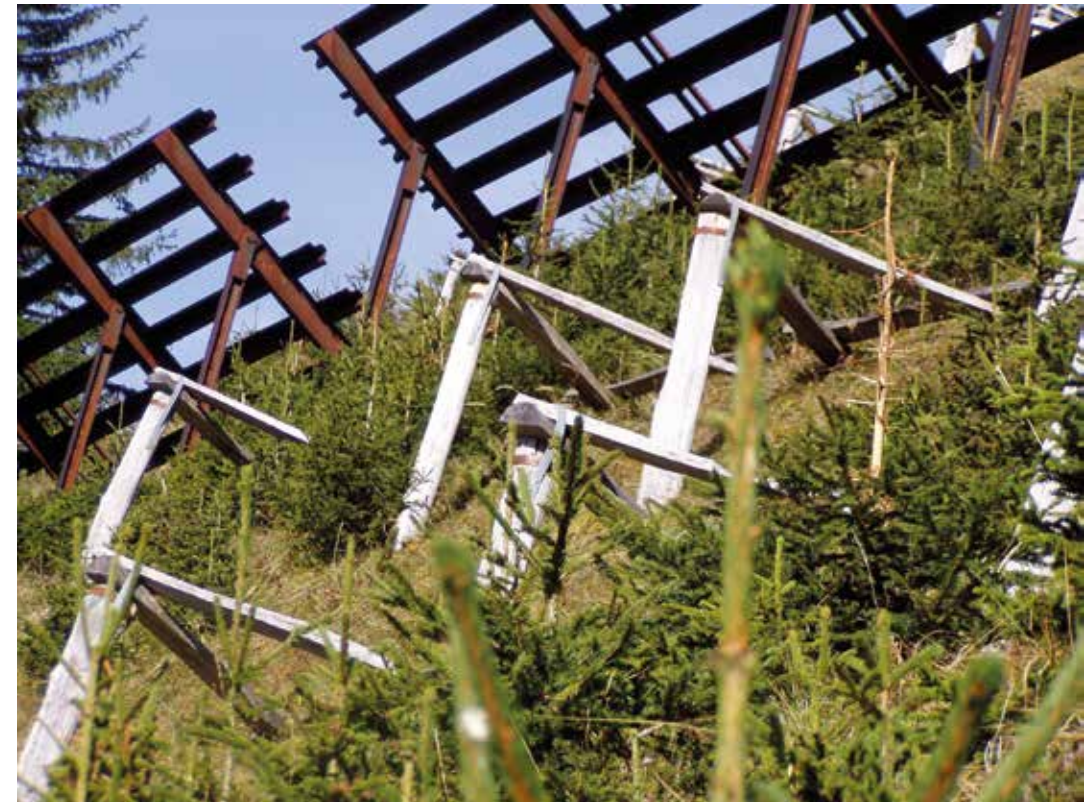
Fig 1: High-elevation afforestation in an avalanche starting zone, controlled by snowpack-stabilizing and anti-gliding structures. Forest can take over the functions of the technical measures in the long run.
