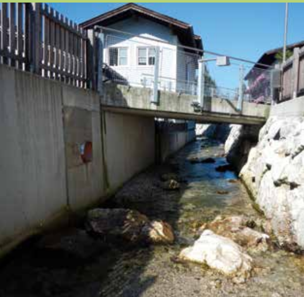
Fig. 3: Torrent channel types with discharge and flow velocity measurements
