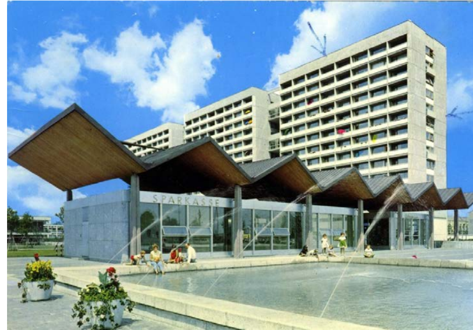
Savings bank's branch in Munich-Fürstenried, built 1961/62
