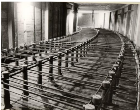
Early attempts at noise damping in Cologne subway construction
