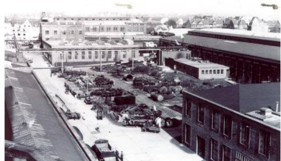
View to Xantener Road, left Land&Sea Cable
