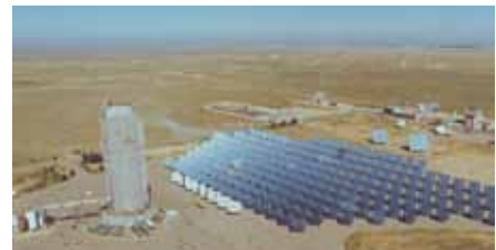
Power Tower von SolarReserve
