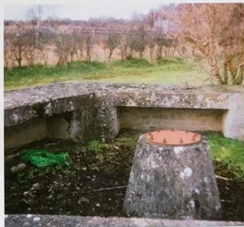
▲ 6-pounder Gun pit showing central pillar gun mounting and moulded ammunition 'lockers'. On Marcham-Frilford crossroads (442971).
