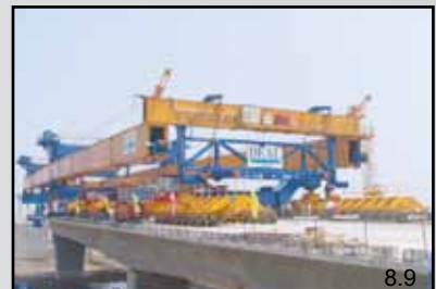
8.9 Bridge & tunnel construction
