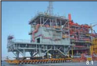
8.1 Offshore & Plant Construction
