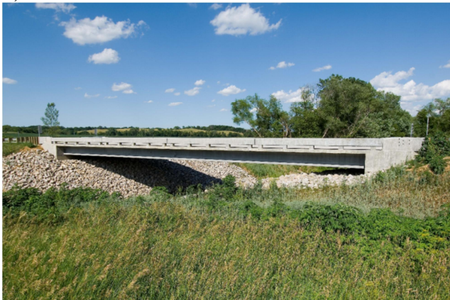
c) Wapello County Mars Hill Bridge
