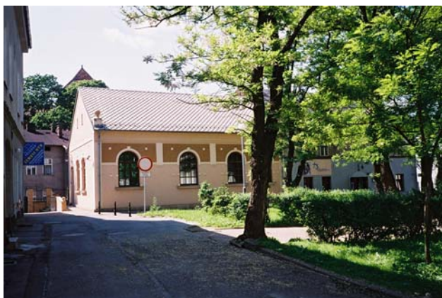
Phot.41. Oświęcim, ks. J.Skarbka Square. The Auschwitz Jewish Center and the Chevra Lomdei Mishnayot Synagogue. View towards the west
