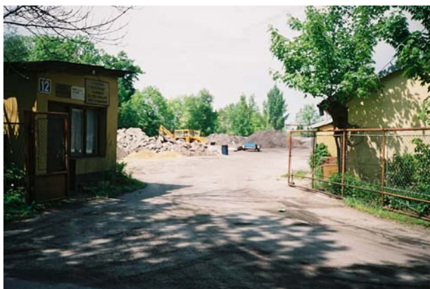
Phot.28. Oświęcim, Leszczyńskiej Street. "Bauhof" premises - former KL Auschwitz construction materials yard (now Road Management). View towards the north-west direction
