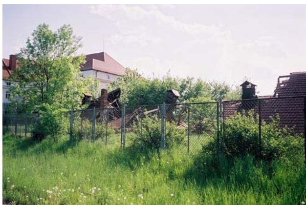
Phot.26. Oświęcim, Spółdzielców Street. "TWL/HWL" - the former SS economic and store base. In the foreground - decaying KL Auschwitz potato stores. View towards the south-west
