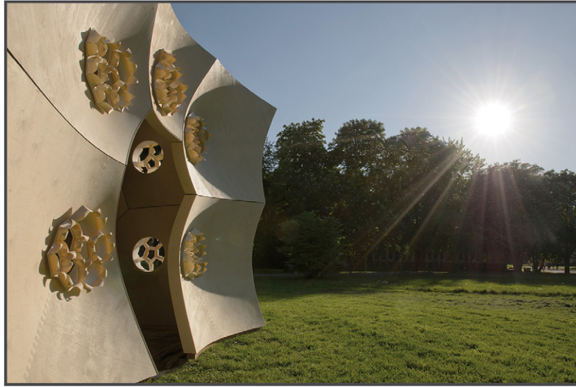
Fig. 20. HydroSkin Pavilion. Decentralized response of elements due to localized changes (solar radiation). Elements not yet exposed (top and bottom right) still partially closed before global RH drops or a localized change takes place due to exposure to the morning sun.
