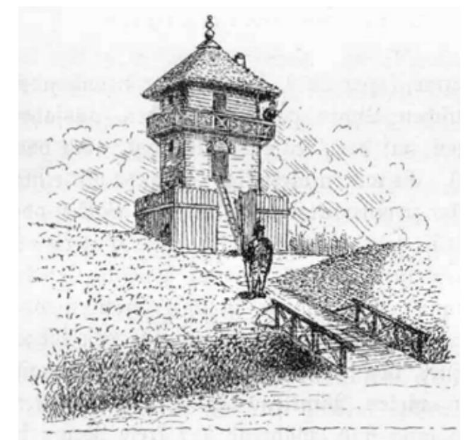
Fig. 2 - Reconstruction of a watchtower at the Odenwald Limes with rampart and moat (Schulze 1912, 40)
