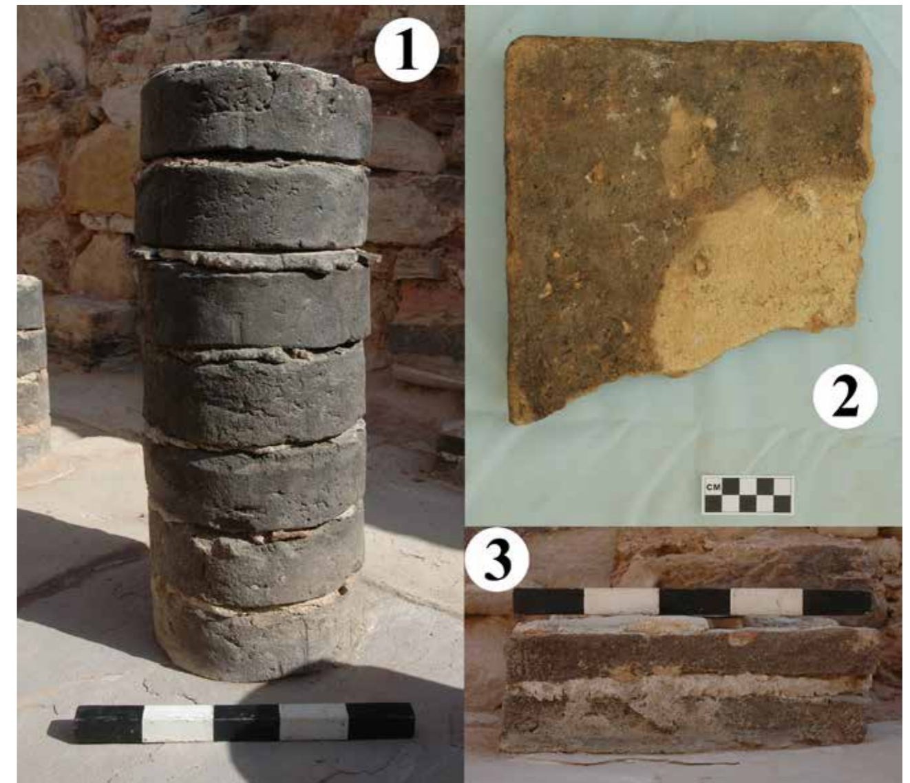
Fig. 3 - Bricks from the praetorium hypocaust system. 1. In situ stack of circular bessales . 2. Pedalis showing shadow of circular bessalis on which it was placed. 3. In situ stack of small rectangular bricks. (Humayma Excavation Project)
