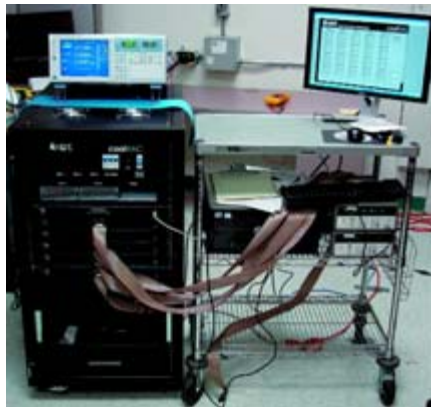
Picture 1: coolRAC Demonstration System
