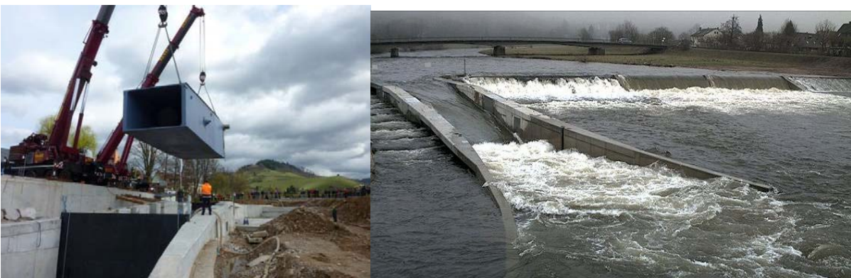
Figure 6: Lowering of the powerhouse and completed hydropower plant in Gengenbach
