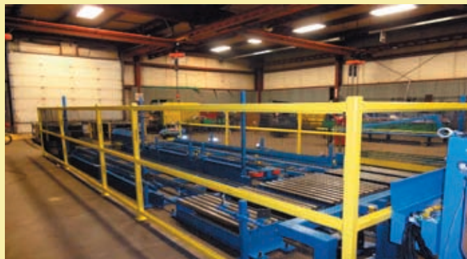
Complete in-house system set-up and testing prior to shipment.
